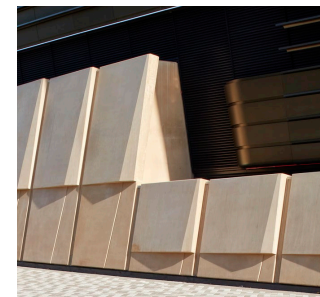
FT06 Concrete walls with varying panel types
