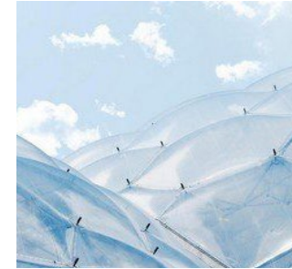
RT01 ETFE roof skin with hybrid steel and timber structure
