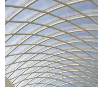
RT01 ETFE roof skin with hybrid steel and timber structure
