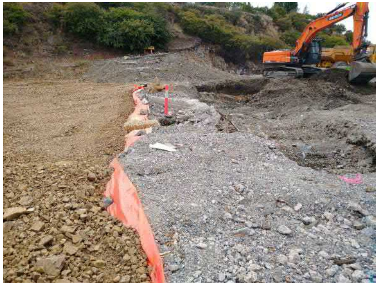
Plate 2 Liner on the Western Boundary of the Telecommunications Cable
