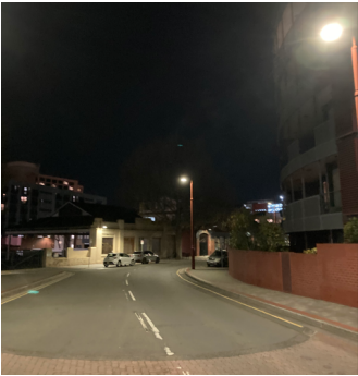
Collins St: Lighting levels ranged from 3 to 30 lux. Lighting is provided by pole mounted luminaires, which appeared to be LED.
