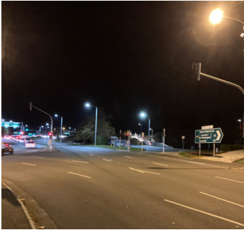
Tasman Hwy: Lighting levels ranged from 10 to 50 lux. Lighting is provided by pole mounted luminaires, which appeared to be metal halide or high pressure sodium lamps.
